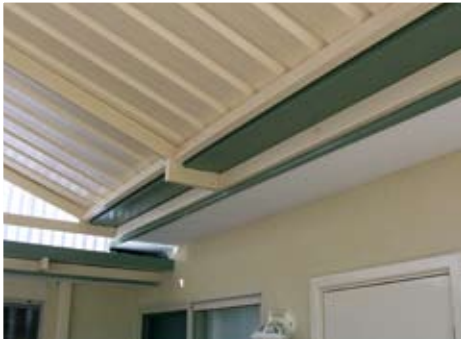
Rafter brackets filled to all patio
